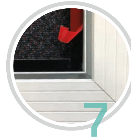
Remove red backing from tape
